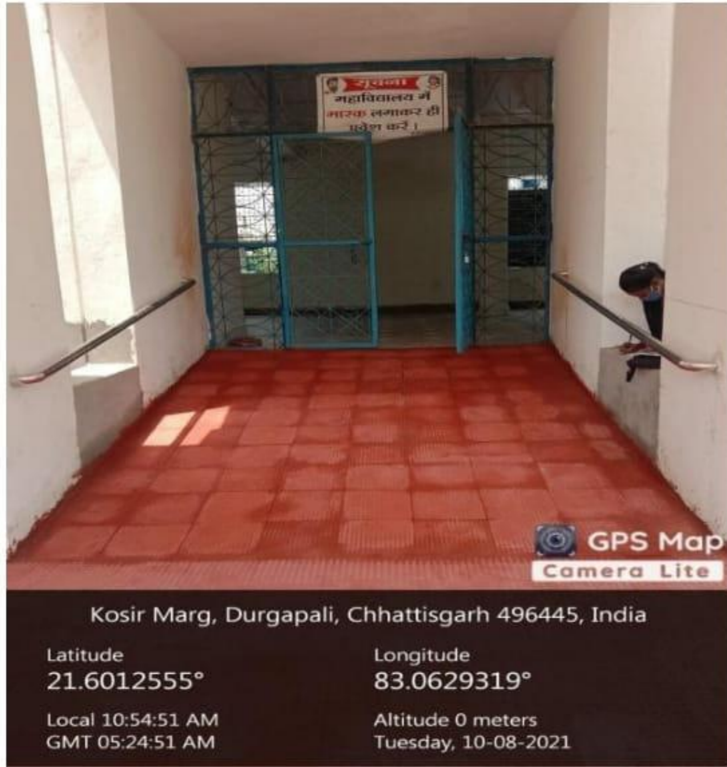
Photograph's of Ramp
